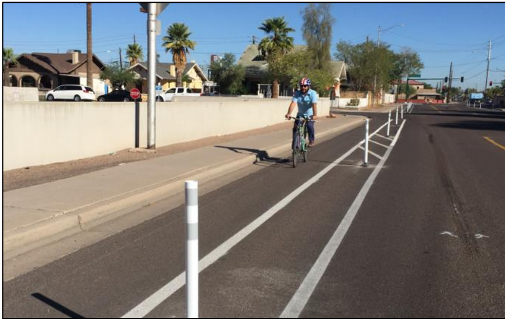
Protected Bike lanes on 15th Avenue from Jefferson to Van Buren Streets.
