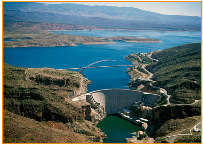
FIGURE 10. ROOSEVELT DAM (SOURCE: BUREAU OF LAND MANAGEMENT)
