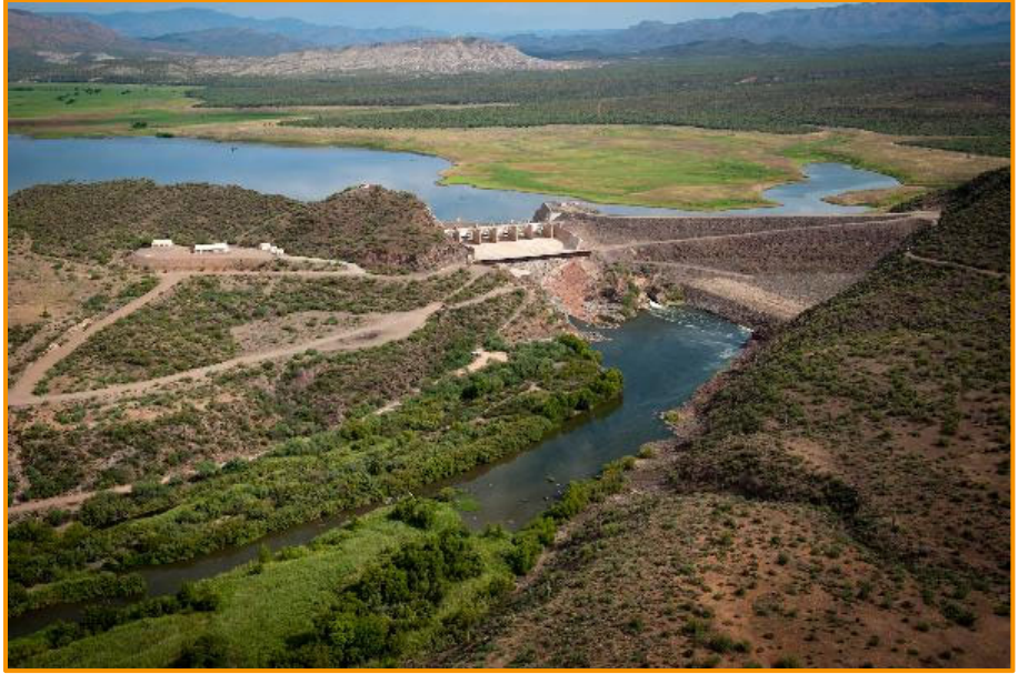
FIGURE 14. HORSESHOE DAM (SOURCE: BUREAU OF RECLAMATION)
