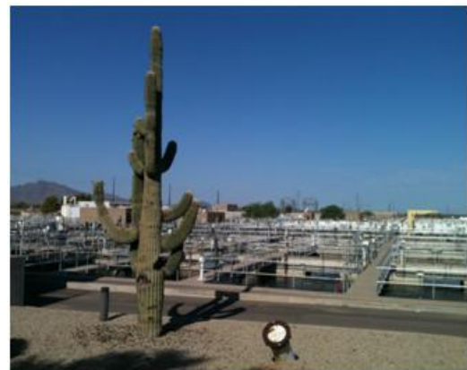
91 st Avenue WWTP Process Basins
